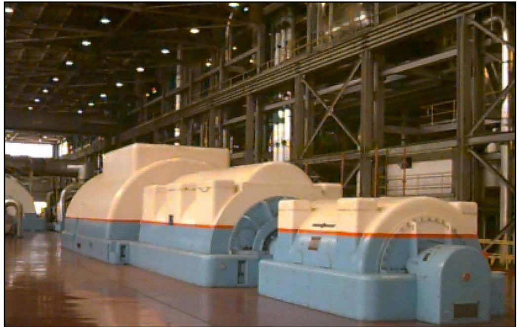
General Electric 680MW turbine
