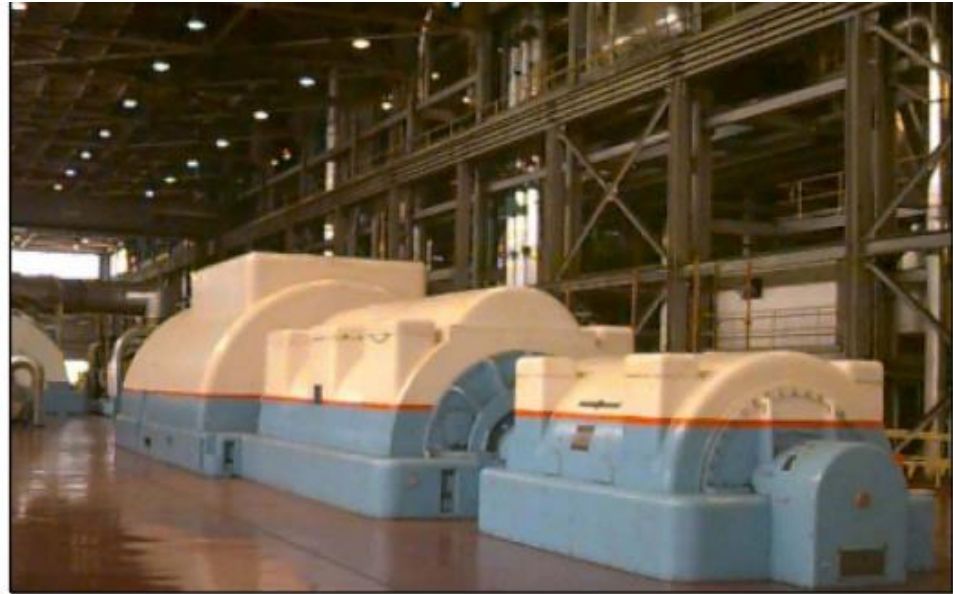
General Electric 680MW turbine
